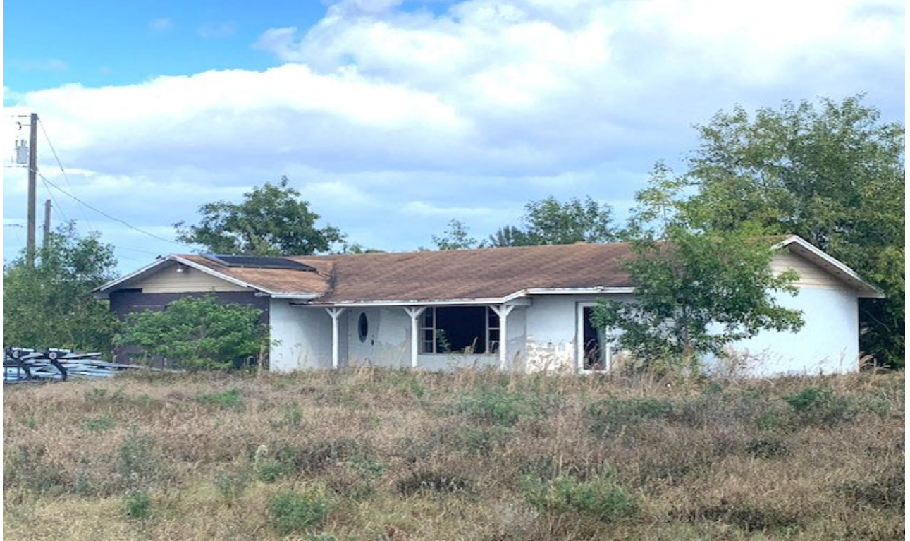
SOUTH & WEST ELEVATIONS OF ABANDONED RESIDENCE ON SITE
