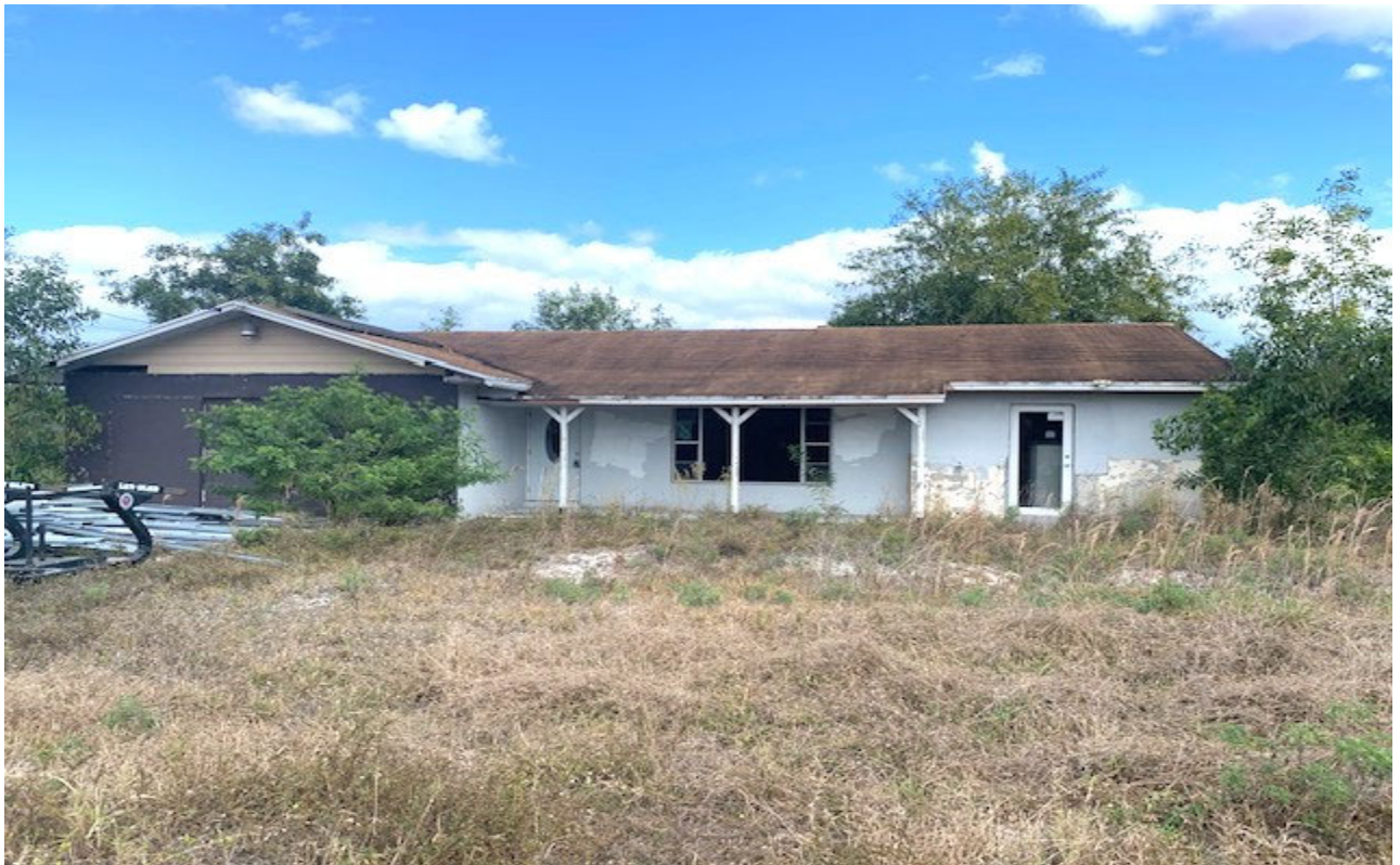
WEST ELEVATION OF ABANDONED RESIDENCE
