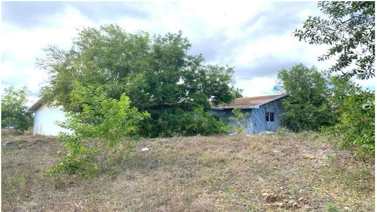
VIEW HOUSE FROM WATER RETENTION AREA LYING SOUTH OF ABANDONED HOUSE
