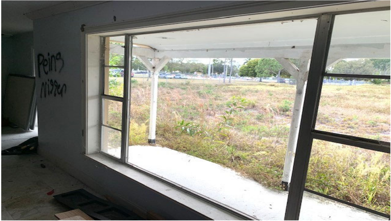
VIEW OF LARGE FRONT WINDOW WITHOUT GLASS
