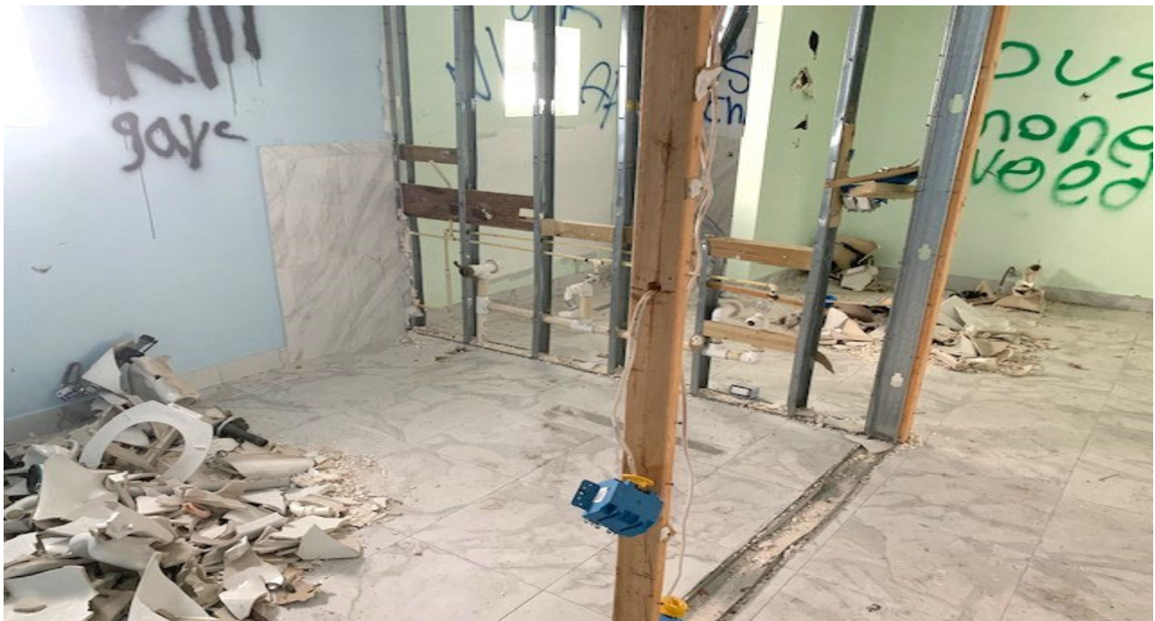
VIEW OF DEMOLISHED BATH AREA OF RESIDENCE
